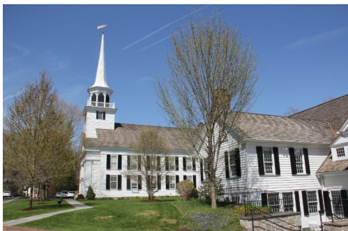
Wilton Congregational Church $2,500.00 for repairs at one of our
